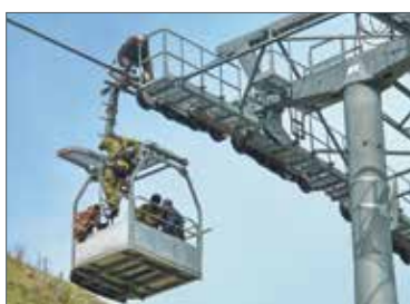
Cable car construction
