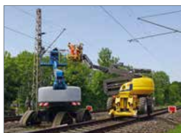
Construction of contact lines
