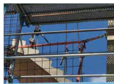
Positioning of loads
