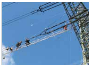
Overhead line construction
